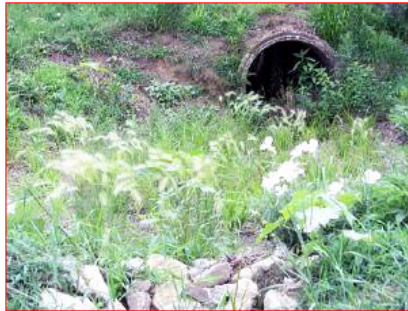
Garden outside drainpipe
