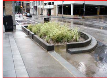
Curb garden to collect runoff
