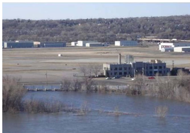
St. Paul Airport at flood stage 19.8 feet. Note floodwalls at water's edge.
