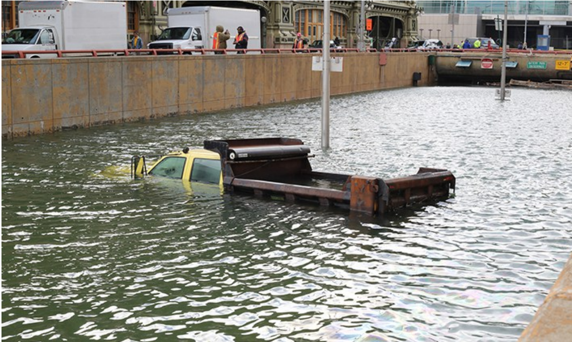
Flooded Battery Park Tunnel after Hurricane Sandy. Photo credit: Timothy Krause /Creative Commons.
