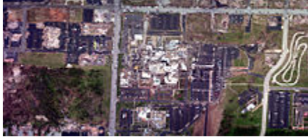
Aerial view of the St. John's Regional Medical Center campus
