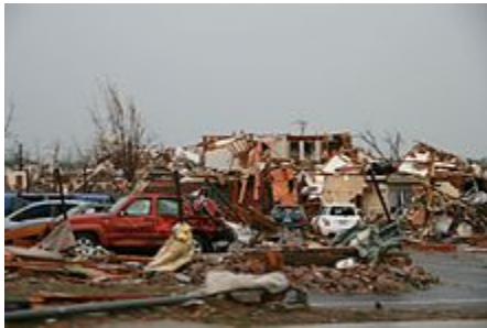
Destroyed area in the tornado's damage path.
