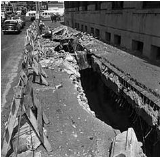
Earthquake damage outside Seattle's Union Station, 1965.
