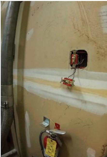
Images: Mechanical Room light switch with missing cover and exposed wires (Left). Example of a damaged cover plate (Right).
