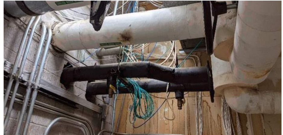
Images: Original basement air-handling unit with blocks supporting isolators and large wall penetration gaps around abandoned pipes.
