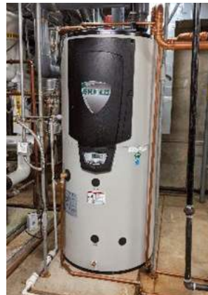
Images: Gas-fired domestic hot water heater next to the heating water boilers with uninsulated domestic hot water piping.
