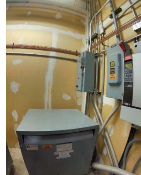
Images: Working space and clearance conflicts in the Electrical Area.
