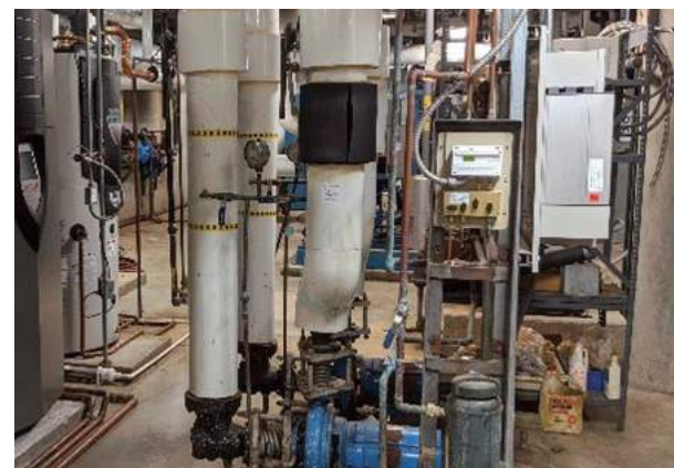
Images: Gas-fired condensing boilers, boiler flue venting, and heating water pumps.
