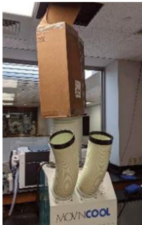
Images: Supplemental cooling unit for instrumentation lab with portable cooler. Walk-in cooler condensation resulting from adjacency to tempered loading area.
