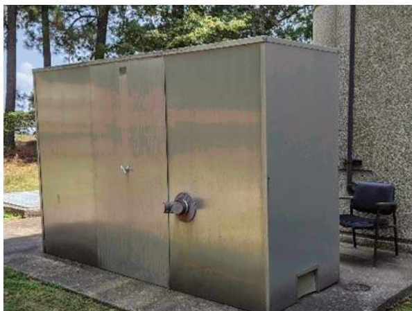
Images: Aboveground backflow preventor in hot box (left), and remote inspector test in mechanical room with drain to floor (right).
