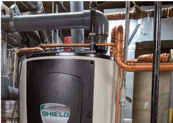
Images: Gas-fired domestic hot water heater next to the heating water boilers with uninsulated domestic hot water piping.
