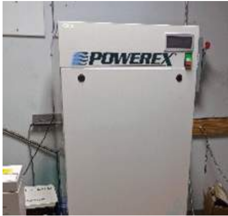
Images: local compressor supporting nitrogen generator
