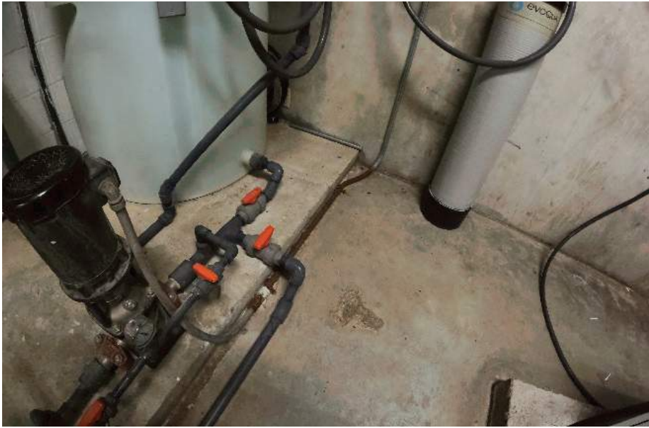
Image: Corroded metal conduit in main mechanical room.
