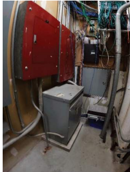
Images: Working space and clearance conflicts in the Electrical Area.
