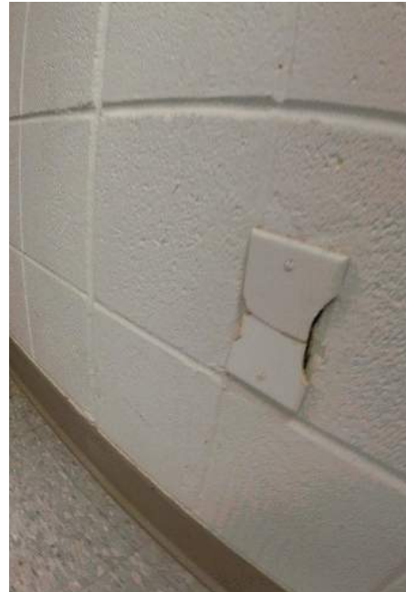
Images: Mechanical Room light switch with missing cover and exposed wires (Left). Example of a damaged cover plate (Right).
