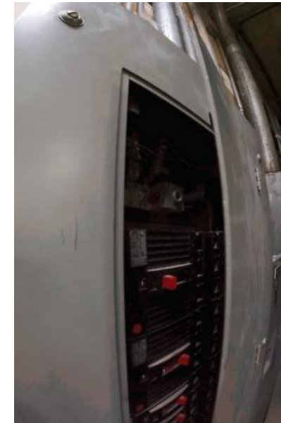
Images: Foreign systems passing through the overhead electrical equipment clearance zones (left). Missing interior cover of a distribution board, exposed live parts (right).
