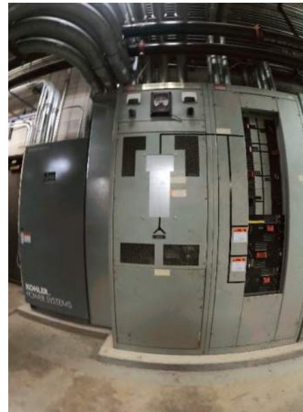
Images: Previous SES with metal panel cover installed (Left). MCC with plastic cover and standard junction box cover installed (Right).
