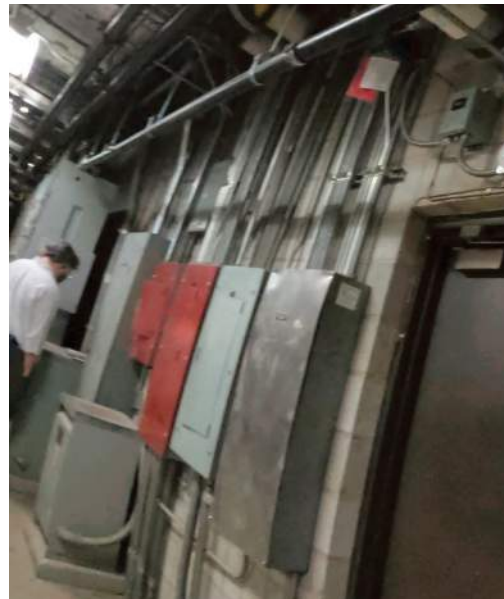
Images: Foreign systems passing through the overhead electrical equipment clearance zones (left). Missing interior cover of a distribution board, exposed live parts (right).
