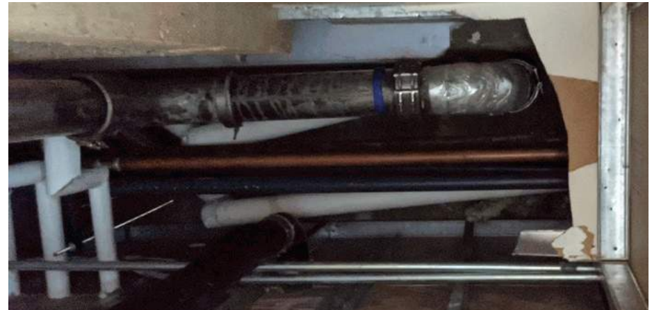
Images: Portions of broken acid waste piping and piping repairs in shaft utilizing cast iron instead of glass.
