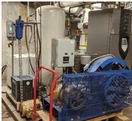
Images: Central compressed air system in the basement (left), and central process vacuum system in the basement (right).
