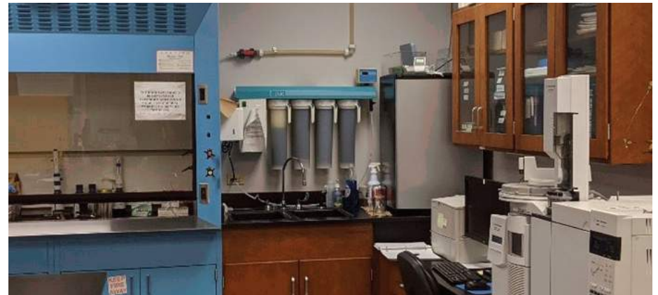
Images: Recirculating reverse osmosis system in the basement complete with water softeners, RO filters, storage tank, and recirculation pump. Local pure water system (bottom) above lab sinks on wall.
