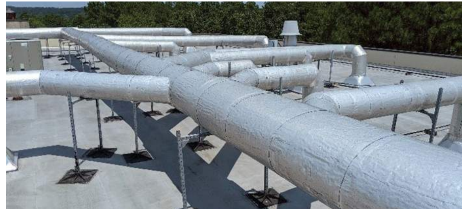
Images: Dedicated outside air heat recovery units with fixed metal plates and general exhaust ducted above the roof. Local fume hood exhaust fans with bypass outside air damper and dilution wind band.
