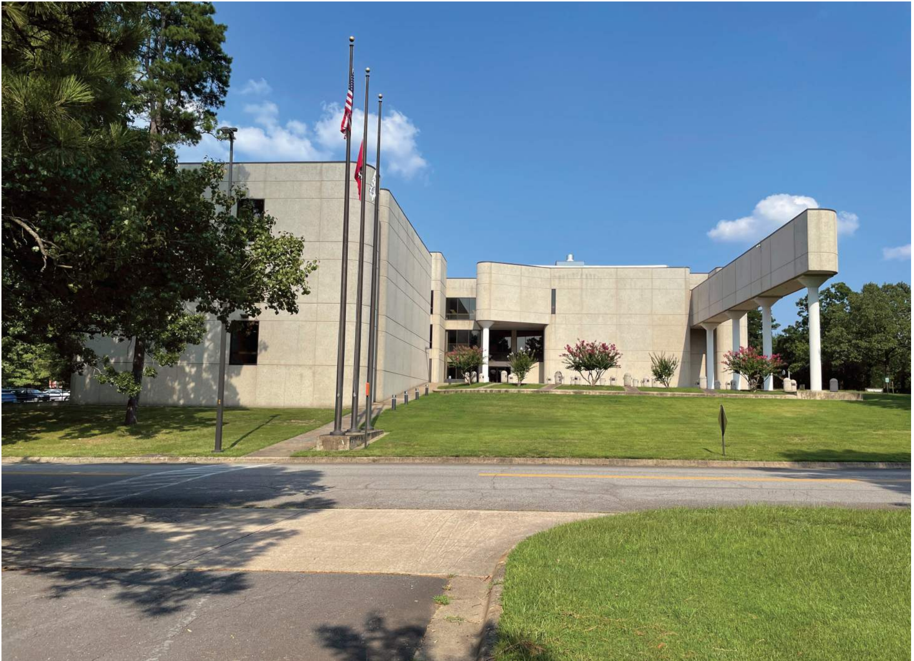
Existing Facility - Exterior
