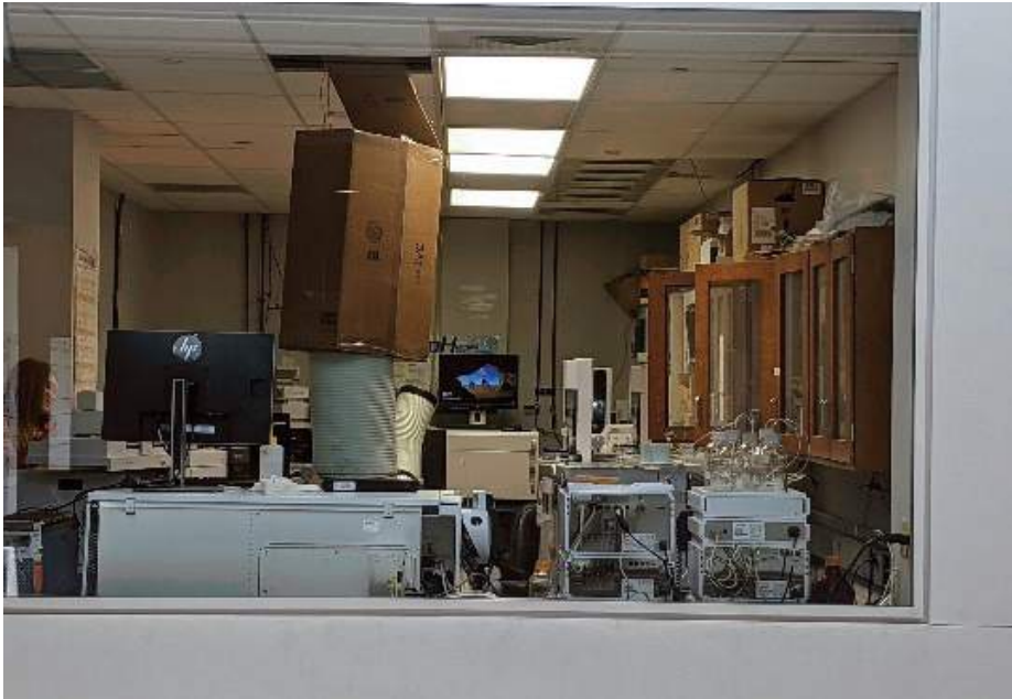
Image: Laboratory support lighting with portable cooling unit and heat rejection "duct".
