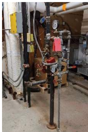
Images: Aboveground backflow preventor in hot box (left), and remote inspector test in mechanical room with drain to floor (right).
