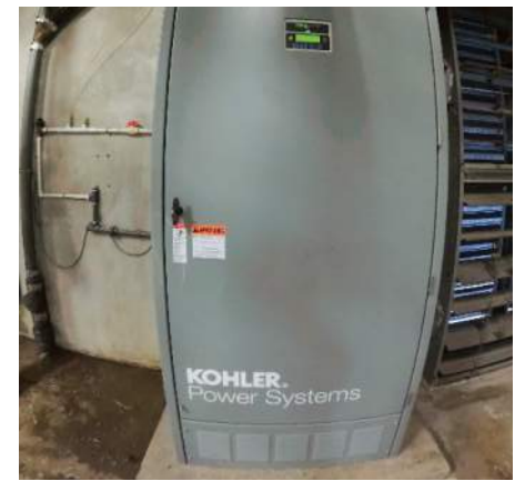
Images: Current ATS units (600A unit on the left).
