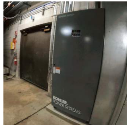
Images: Current ATS units (600A unit on the left).
