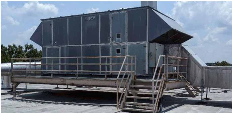
Images: Dedicated outside air heat recovery units with fixed metal plates and general exhaust ducted above the roof. Local fume hood exhaust fans with bypass outside air damper and dilution wind band.
