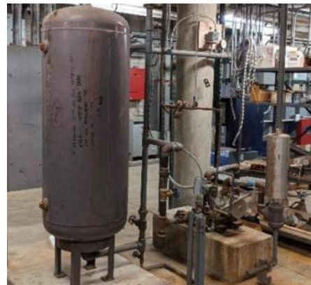
Images: Central compressed air system in the basement (left), and central process vacuum system in the basement (right).
