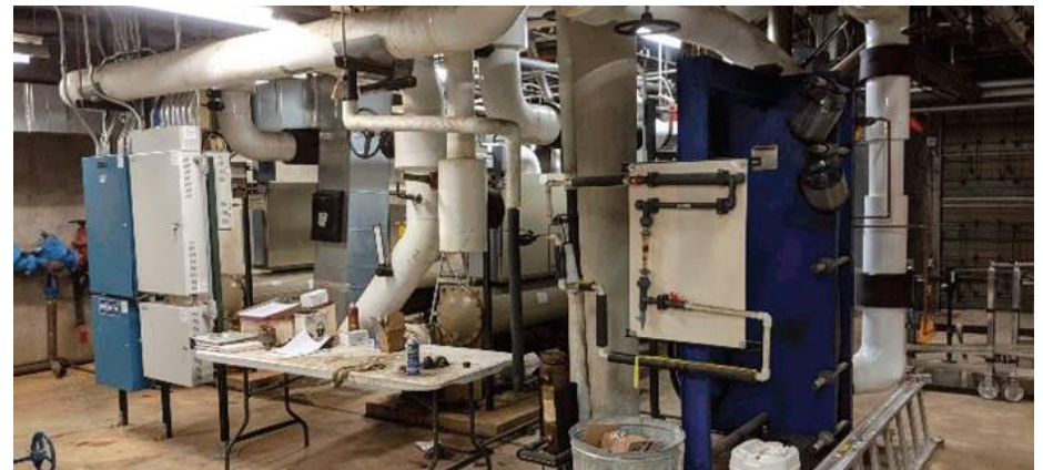
Images: Proximity issues of electrical gear and panels from mechanical, plumbing, and fire protection distribution in central plant.
